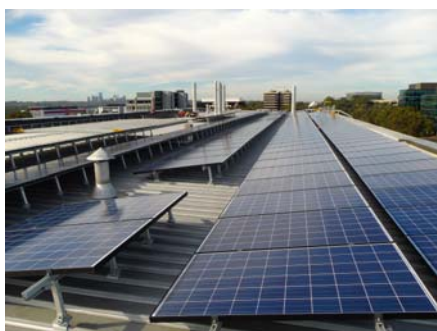
Solar Panels - Sonic headquarters
