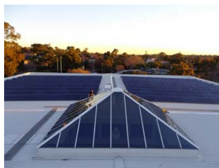
Solar Panels – 95 Epping Road, Macquarie Park
