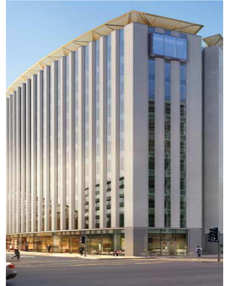
New Sonic UK lab – H2 CY2016 “Halo Building” Euston Road Central London
